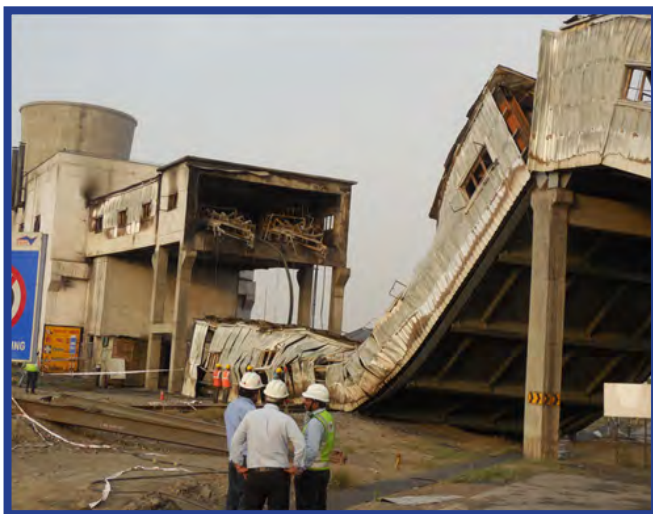
Fig.1: View of damaged conveyor line
