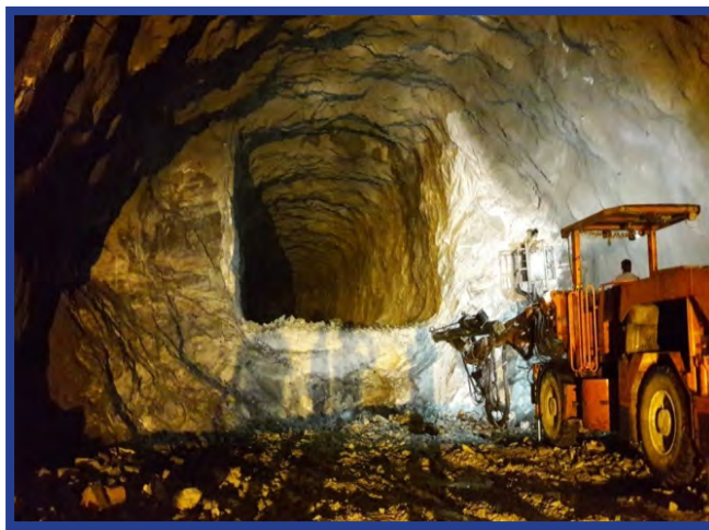
Photo 12: Rock excavation for construction of desilting chamber at Vishnugaad-Pipalkoti Hydroelectric project
