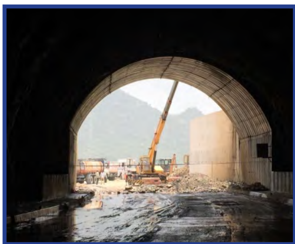
Photo 7: Collapse of slope above Sirohi tunnel portal
