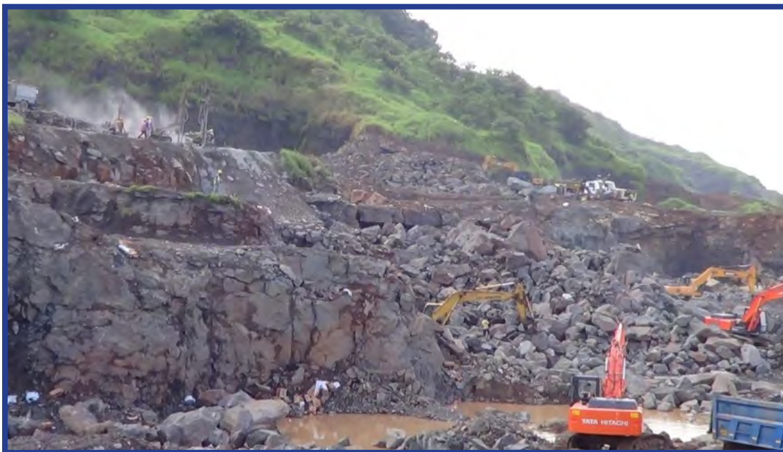
Drilling and mucking operation at Package-III of the Ulwe hill, NMIA.
