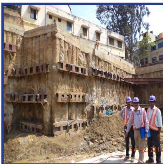
Fig. 5 (b): Rock excavation near sensitive structures at Majestic station of Bangalore Metro Rail Project
