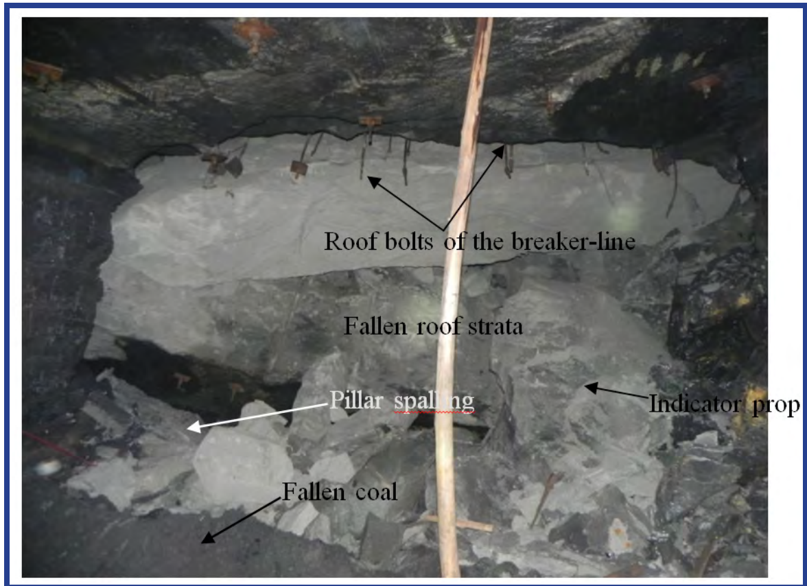
Fig.5: Application of RBBLS (high density of bolts) to resist extension of roof fall ahead of the goaf edge.
