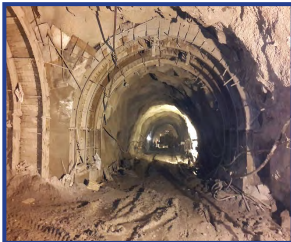
Fig. 3 : Excavation of multiple tunnels at complex geological conditions at Rammam Hydro-electric project-III.
