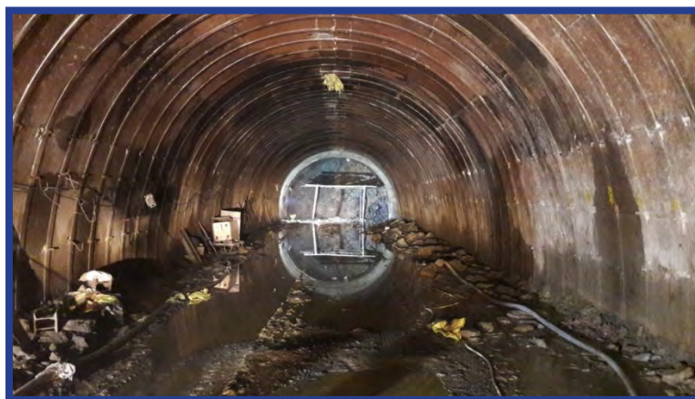
Photo 10: Rock excavation and support design in Saranada railway tunnel on Mumbai-Howrah rail line
