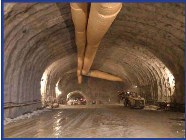
Photo 3: Inside view of ventilation cavern showing lattice girder support covered with shotcrete, Z-Morh Project, J & K (Source: ITNL, Gandhinagar)
