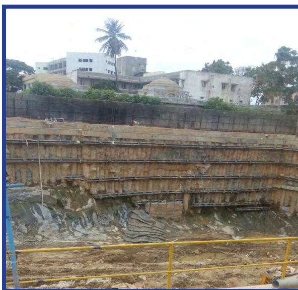
Fig. 5 (a): Rock excavation near critical structures at City Market station of Bangalore Metro Rail Project
