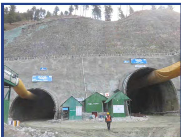
Photo 1: West portals of Escape and Main Tunnels of Z-Morh Project Under Construction on Srinagar-Sonamarg Highway, NH-1 (Source: ITNL, Gandhinagar)
