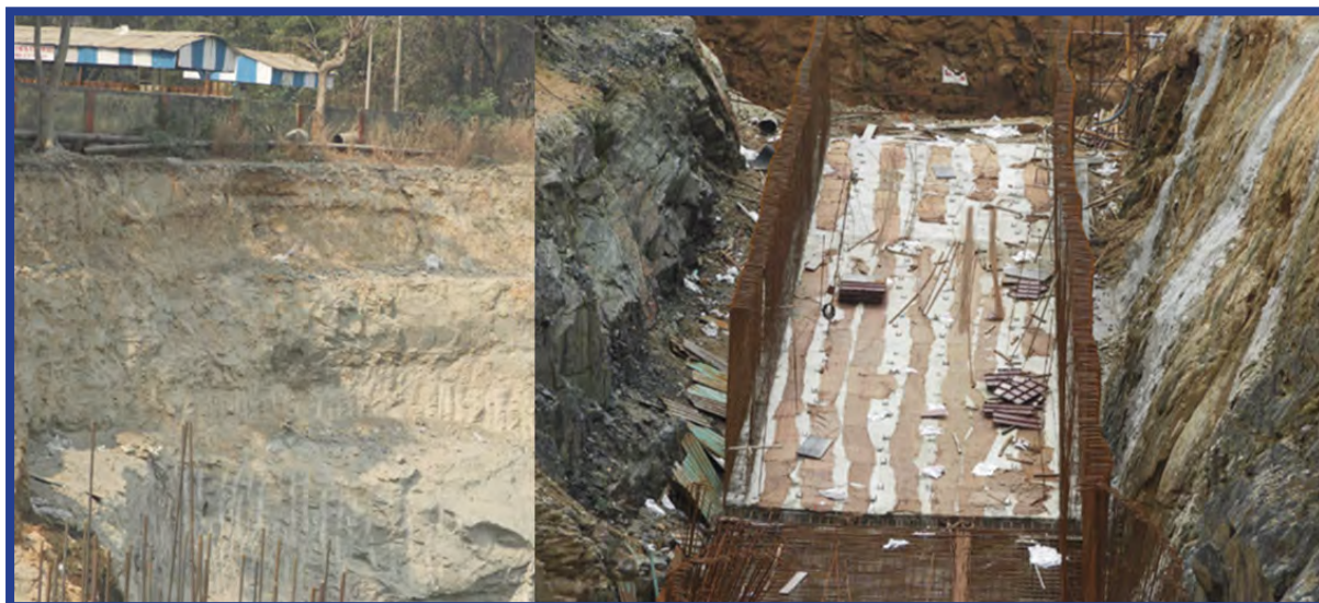
Controlled blasting carried out within 20 m from active Petrol Pump, Wagon Tippler Complex TSTPS, NTPC, Kaniha
